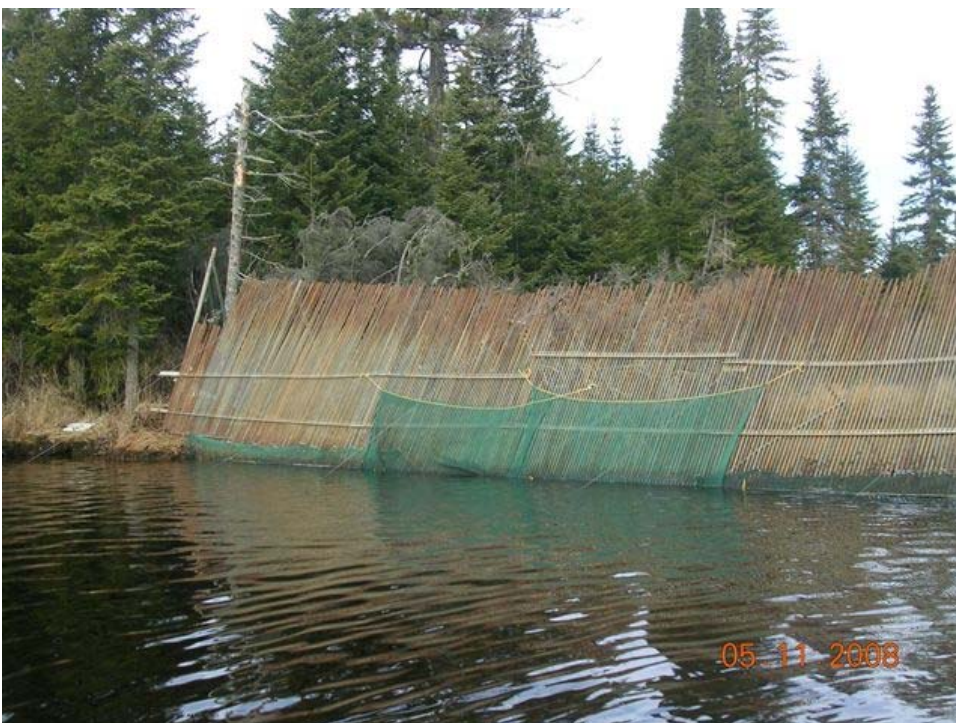
Containment fence at lake outlet.
